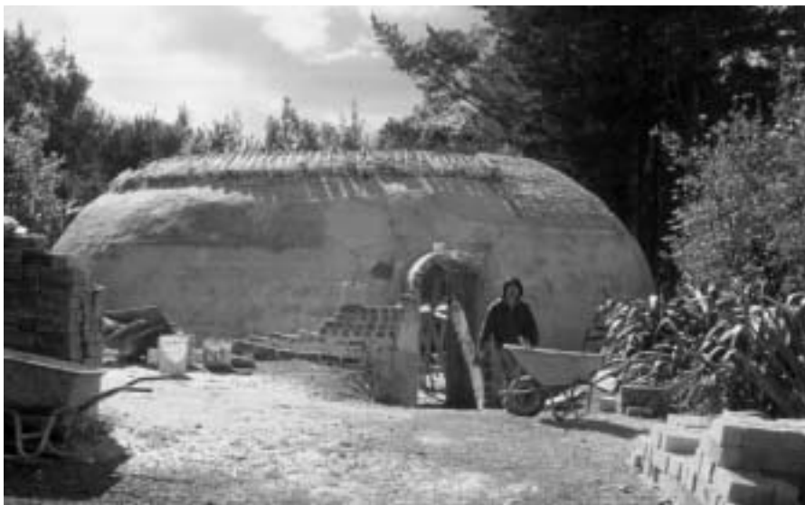
We built a dome-shaped building for an old Buddhist monk.
